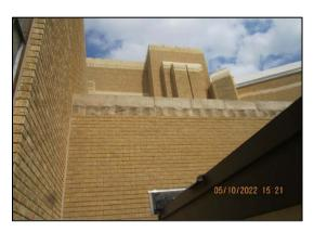
(5) On the West Elevation at the 1970s addition, there are 2 pre-cast stones that shall be replaced.
