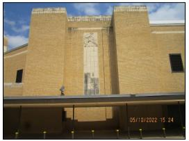
(3) All stone-to-stone joints shall have all old sealant removed. Once complete, all skyward facing joints shall have new silicone sealant installed. All remaining stone-to-stone joints shall then have new Type "N" mortar installed, matching original mortar as closely as possible in color and appearance.
