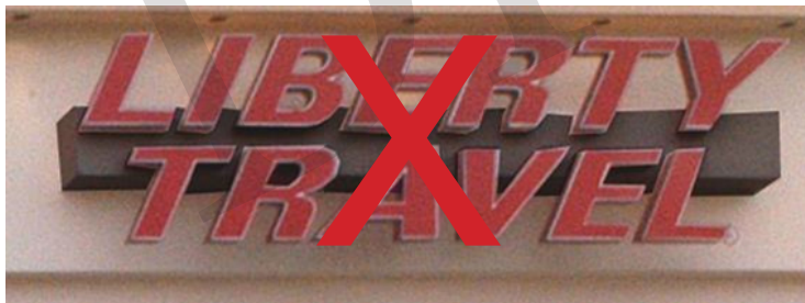
Above: Raceways less than 50% of the height of the letters and not painted to match the background are not allowed.
