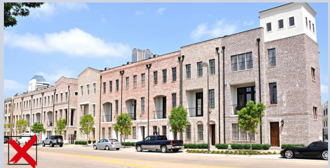
The lack of stepbacks in this townhome project results in a tall, flat facade with a more bulky appearance.
