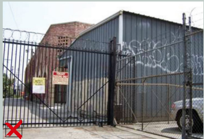
Blocked alley access.
