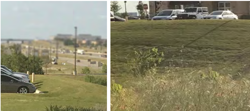
BERM IS AT A CONSISTENT HEIGHT AND DOES NOT USE PLANTING TO ACHIEVE THE REQUIRED PARKING SCREEN
