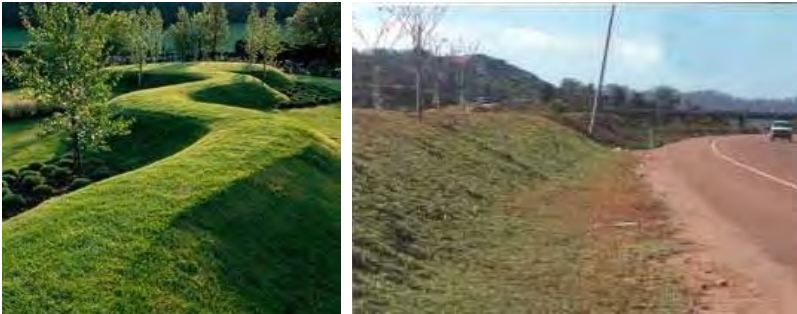
EXAMPLES DO NOT EXPRESS A NATURAL VERTICAL CHANGE IN ELEVATION OVER THE LENGTH OF THE BERM
