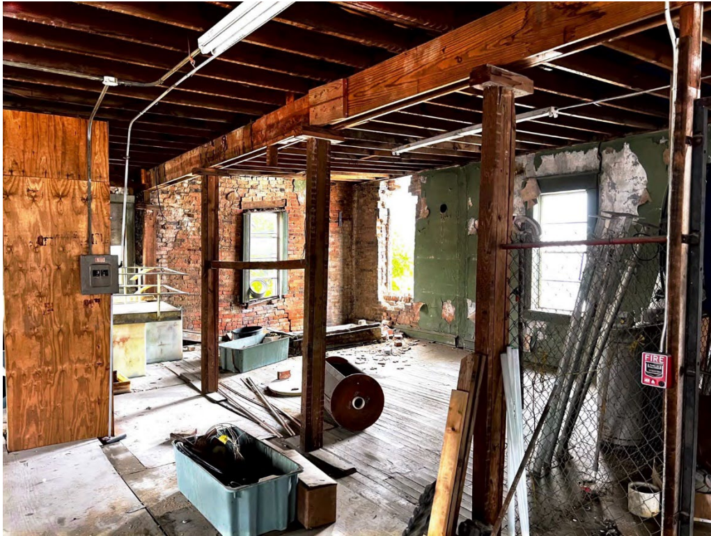
Figure 11. Site photos taken June 7, 2024 before construction
