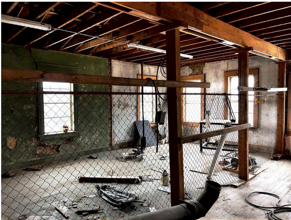
Figure 14. Site photos taken June 7, 2024 before construction
