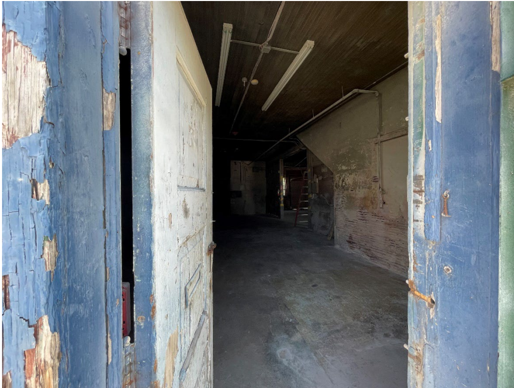
Figure 20. Site photos July 3, 2024
