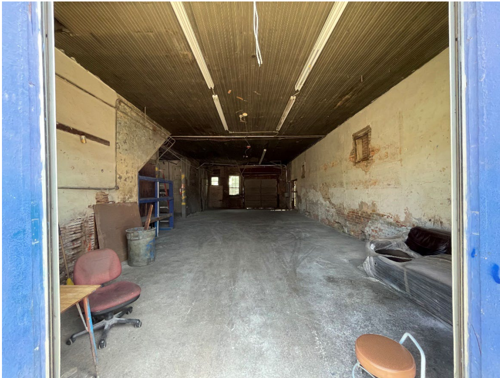
Figure 19. Site photos July 3, 2024
