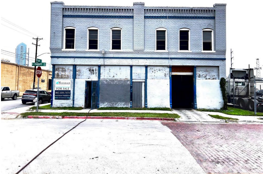
Figure 10. Site photos taken June 7, 2024 before construction
