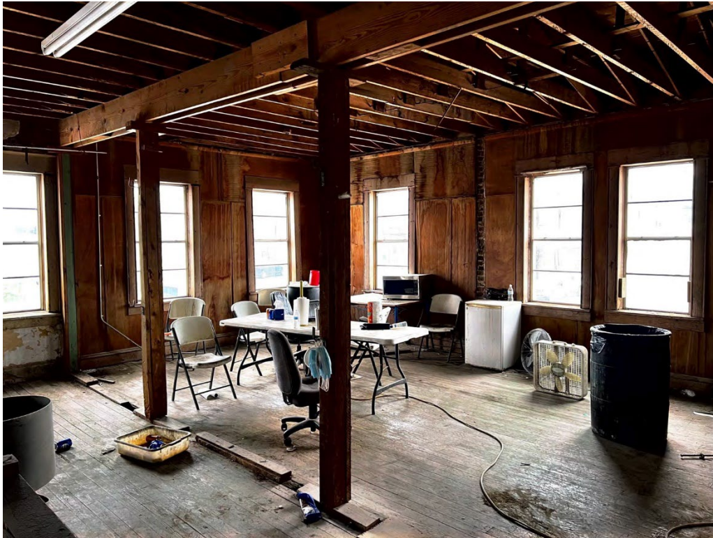
Figure 13. Site photos taken June 7, 2024 before construction
