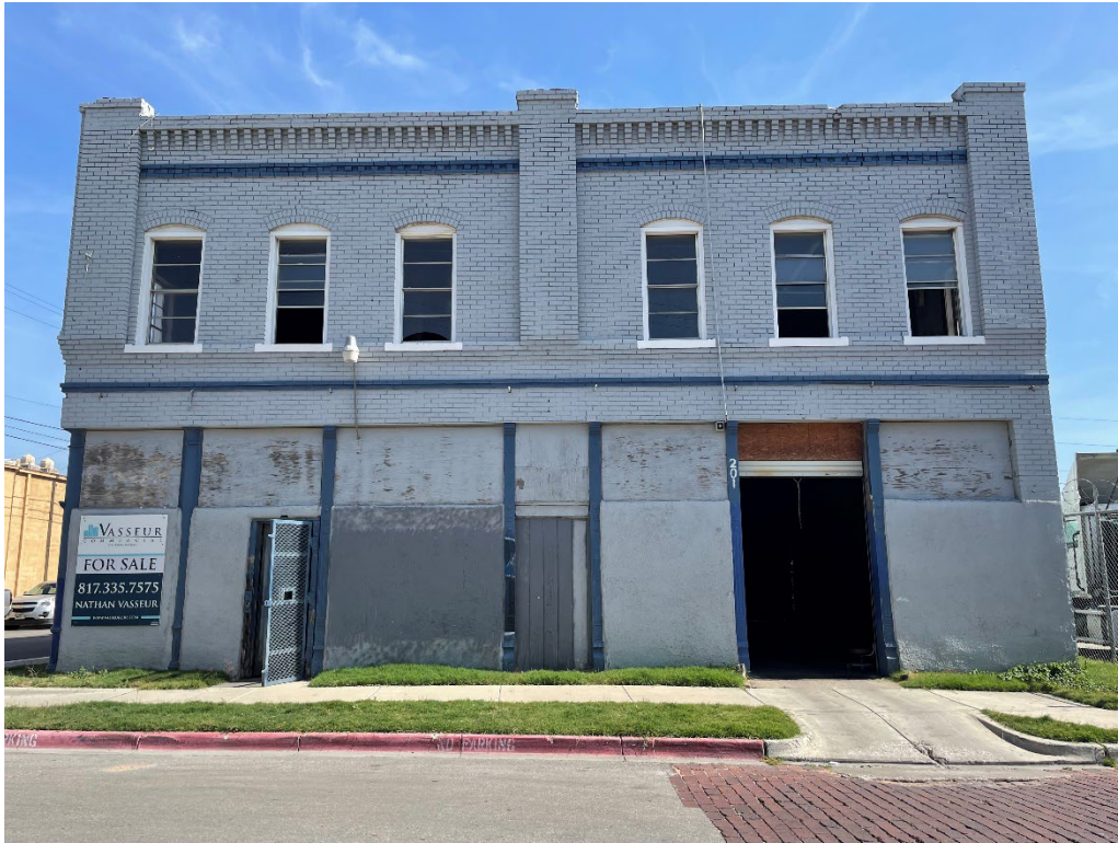
Figure 18. Site photos July 3, 2024
