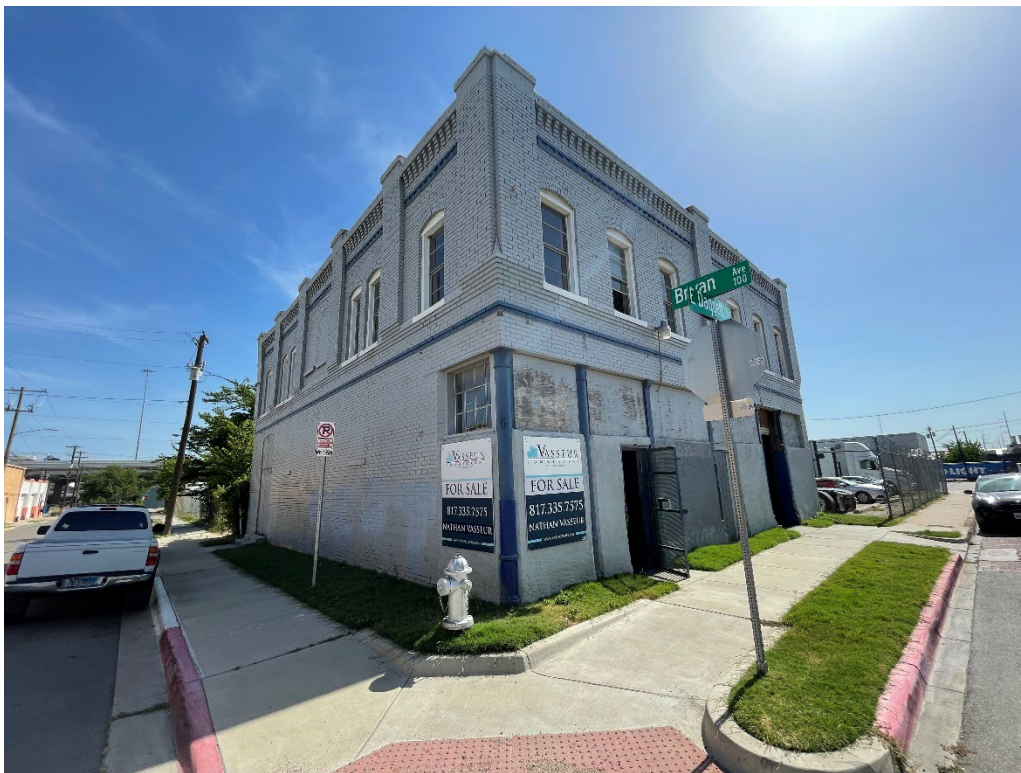
Figure 21. Site photos July 3, 2024
