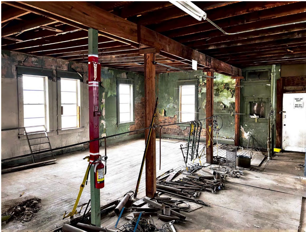
Figure 12. Site photos taken June 7, 2024 before construction
