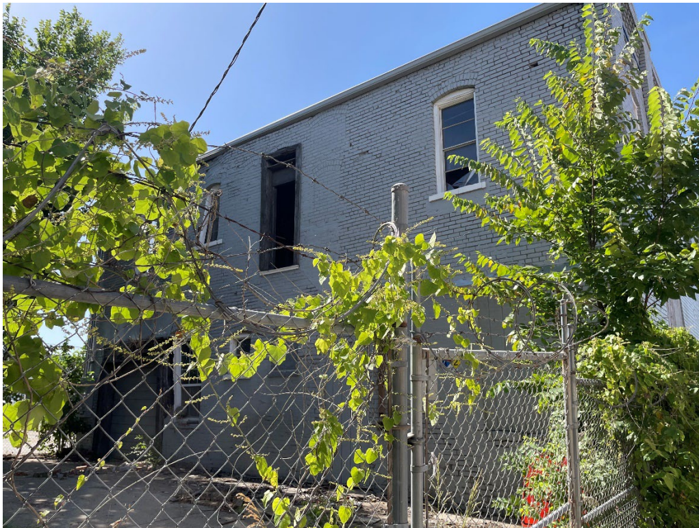
Figure 23. Site photos July 3, 2024, rear.
