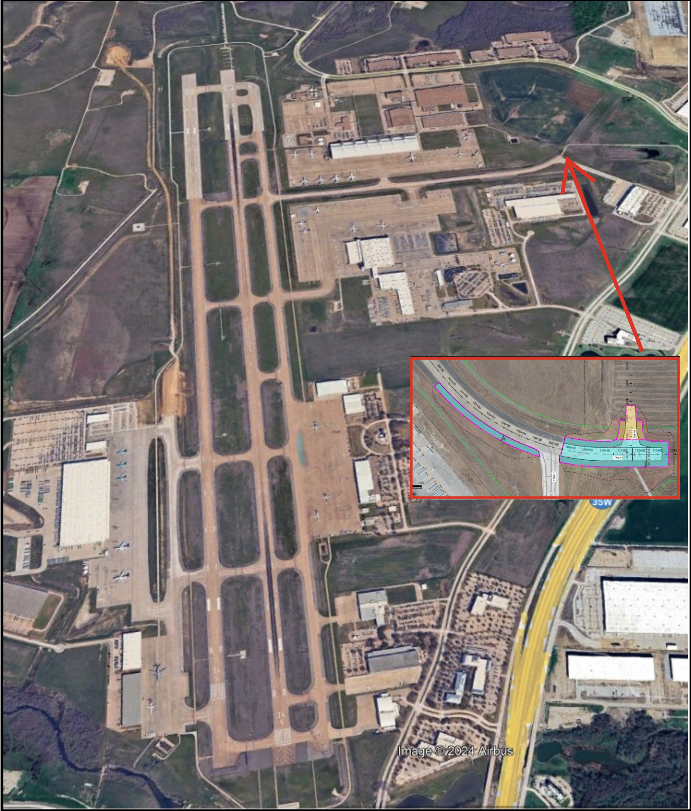
PEROT FIELD FORT WORTH ALLIANCE AIRPORT
