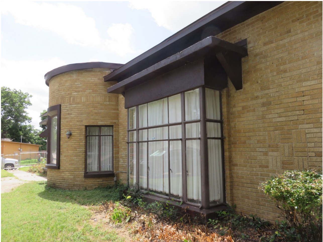
Figure 9: Entrance Bay and west window (2024)
