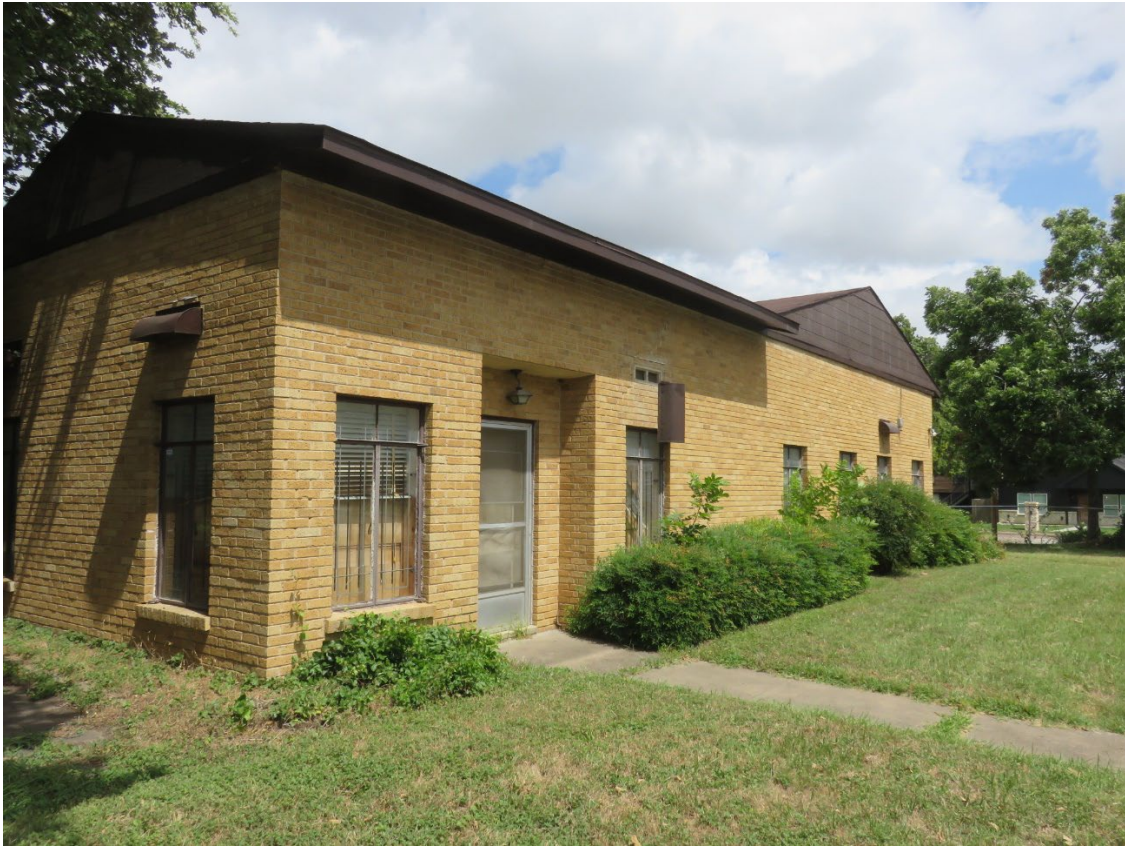
Figure 4: East elevation, looking from S Chandler Dr
