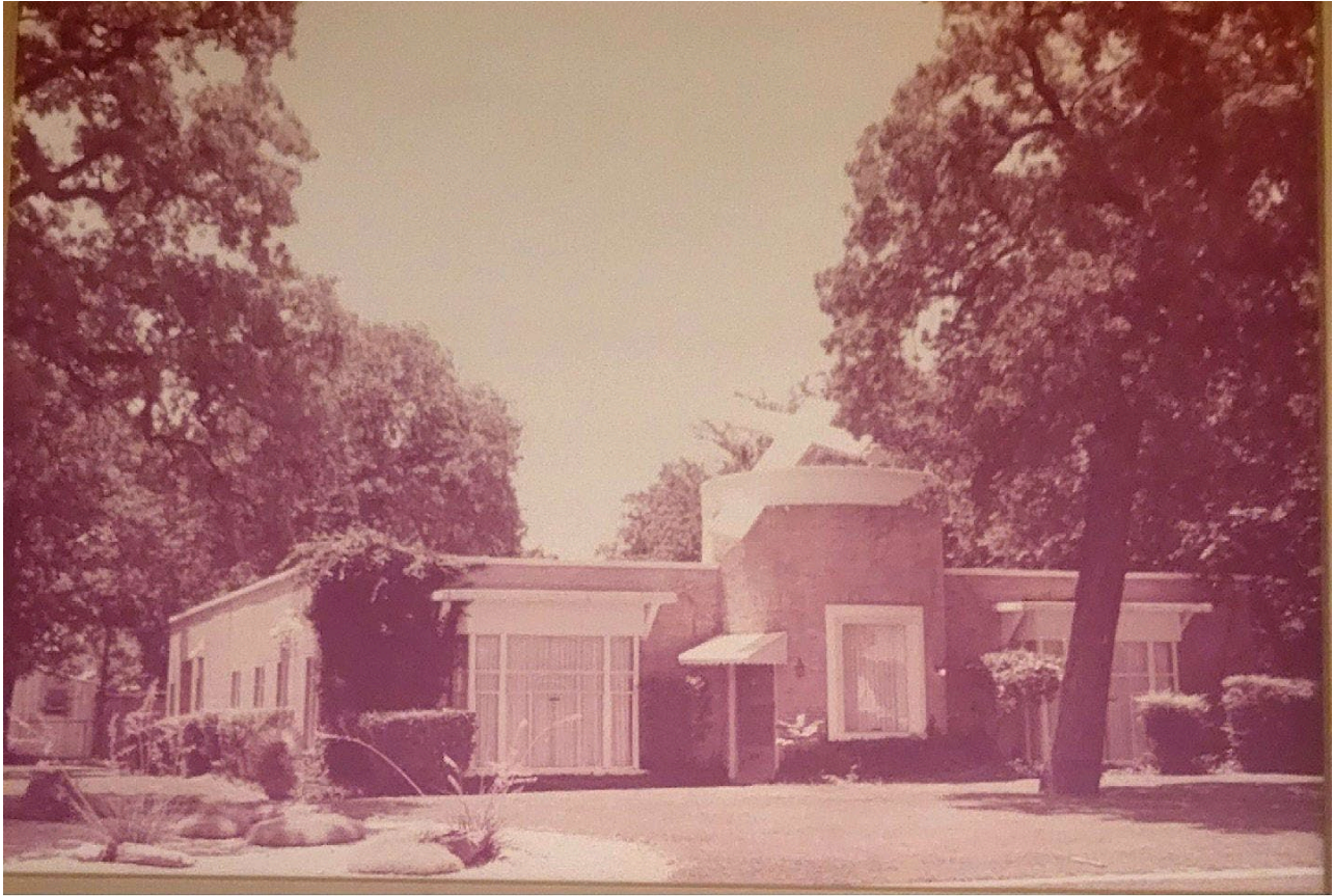
Figure 6: Historic Photo of Headquarters Building (undated)
