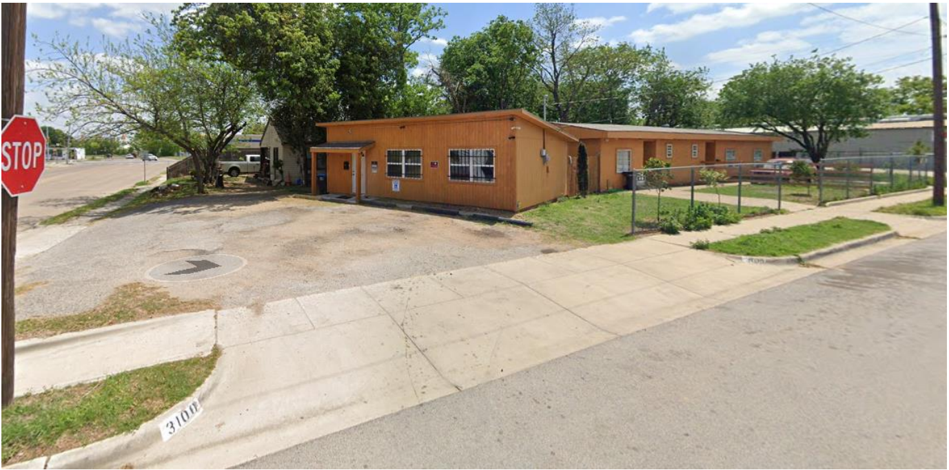
Figure 2- View to the South
