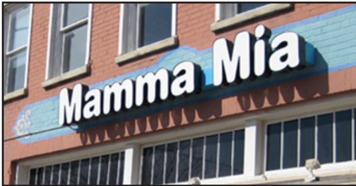
Above: The raceway is painted to match the background.
