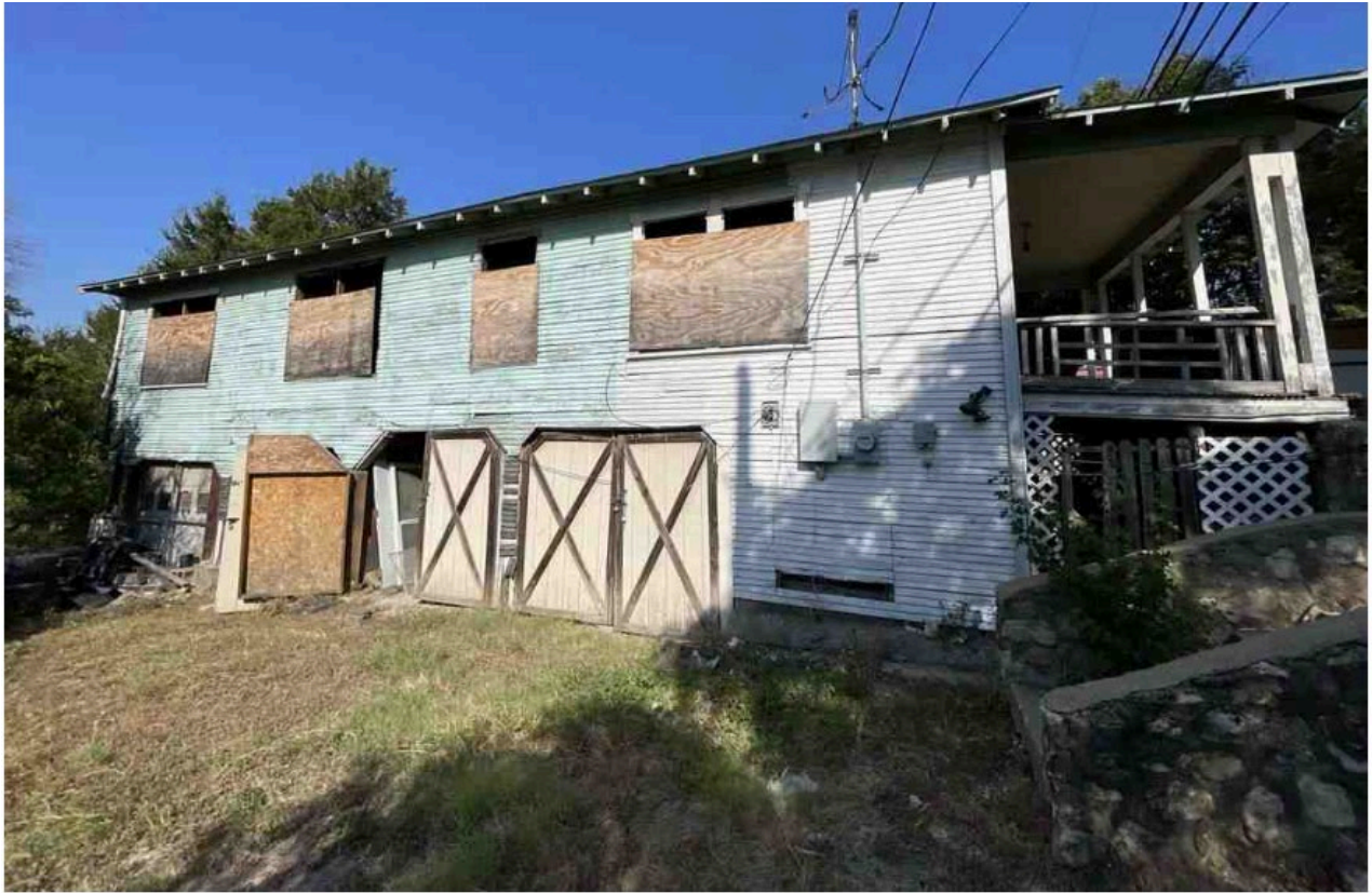
Figure 7. Side of the back house.
