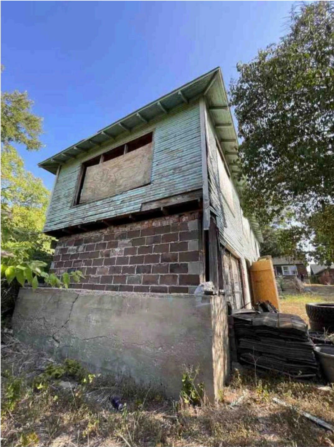
Figure 8. Rear of the back house.
