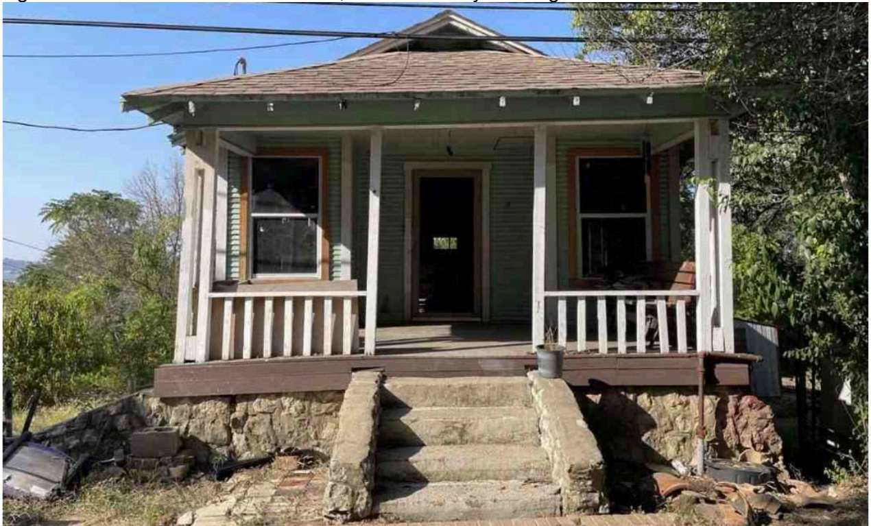
Figure 6. Front of the back house.
