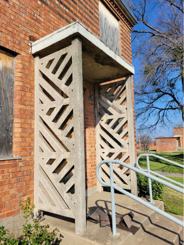
Figure 13 Cast Concrete porch supports
