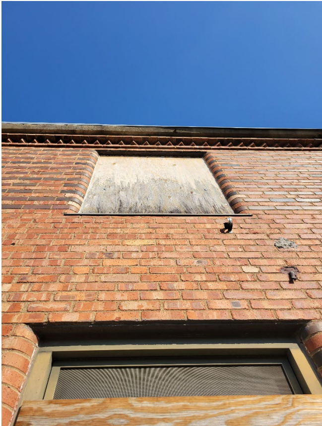
Figure 16 Detail view of curved brick and angled header brick
