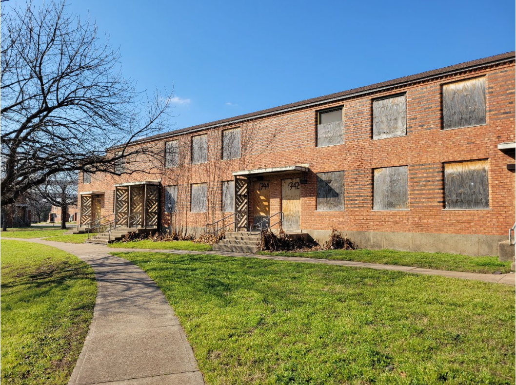
Figure 12 Rear view of 1715-1750 Stephenson St
