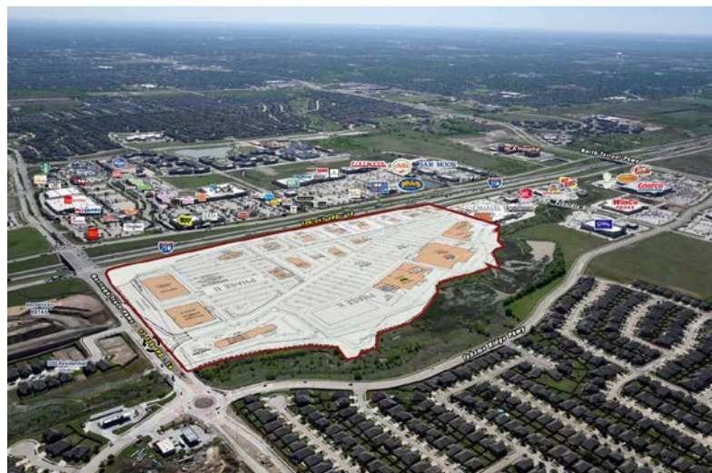
Aerial with development overlay – looking southeast
