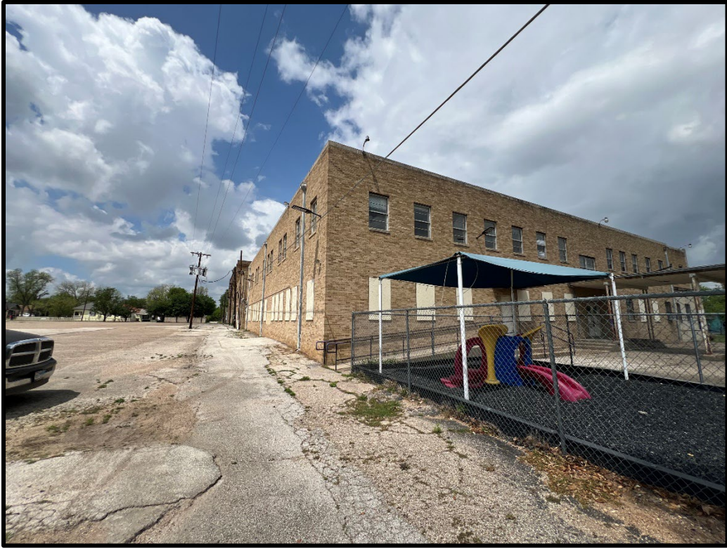
View of building and referenced alley (Facing northeast)
