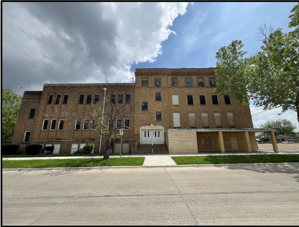
View of building from NW 15 th Street (Facing South)
