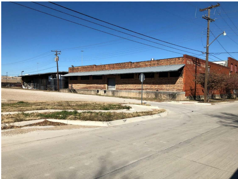
Fig. 5 – Rear or structure. Note the differentiation to common brick and stepped parapet. The south elevation historically fronted on a railroad spur line, now an unimproved section of Jarvis
