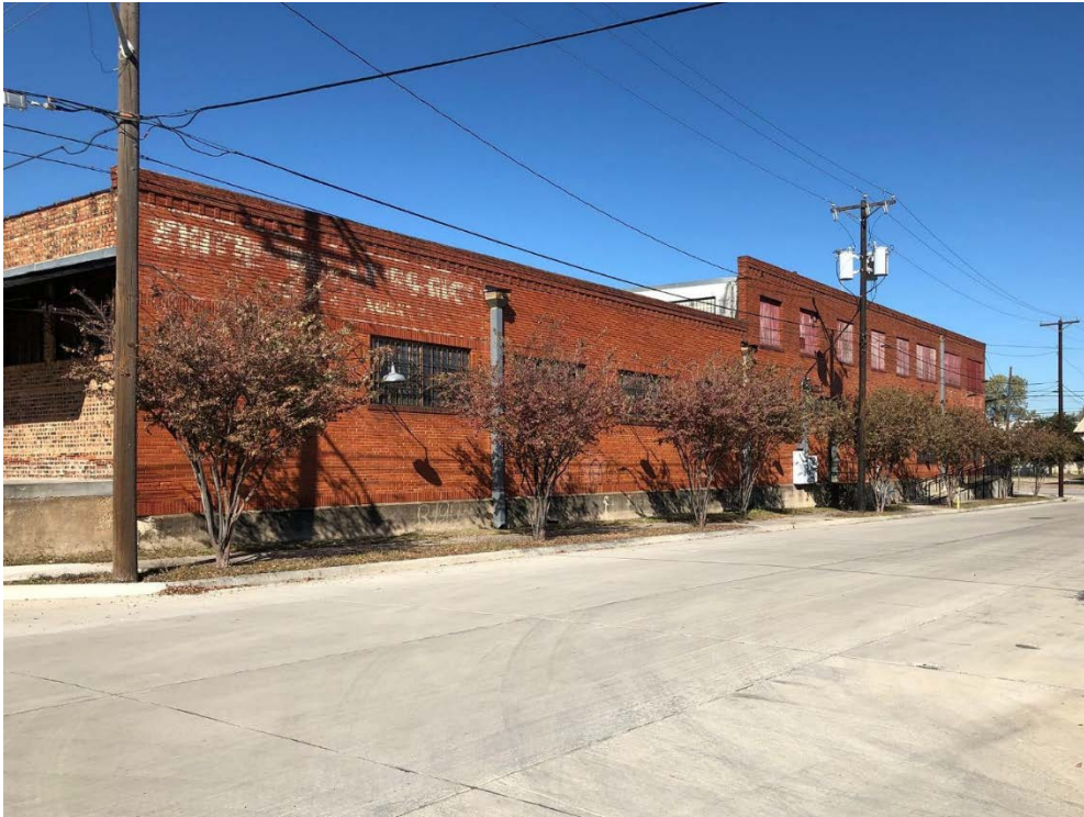
Fig. 4 – Eastern elevation, showing polychrome original masonry. Note that original windows remain behind the boarded up openings on the second floor. Painted-on signs are apparent on the east elevation but are illegible.
