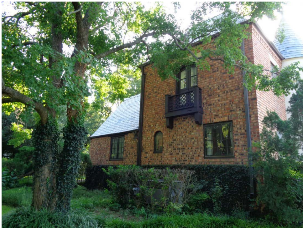
Fig. 7 – Eastern elevation, showing polychrome brick, original multi-light wood windows.
