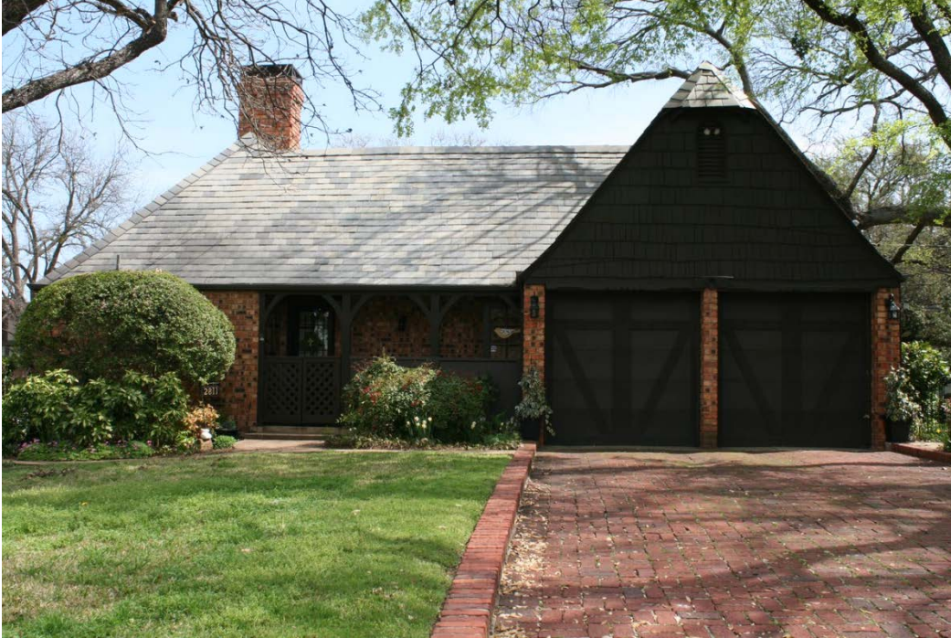
Fig. 8 – Western elevation, showing French Eclectic details such as timber framing, flared eaves, and a clipped gable over the garage.
