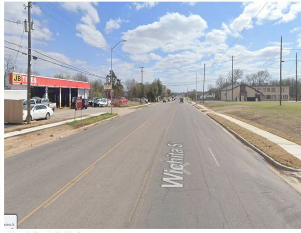
Figure 2-View to the South
