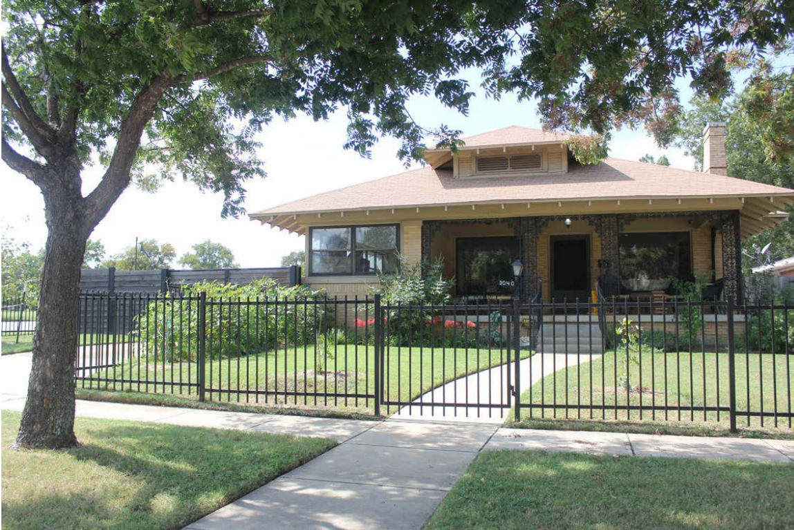
Fig. 4 – 1308 Lincoln Avenue. Note porch enclosure and original masonry column on left of porch.
