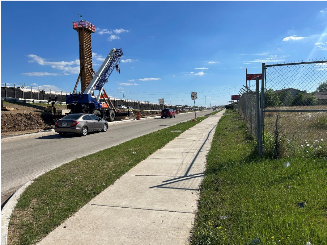
Figure 9. Rights-of-way adjacent to E Loop 820 S FWY Service Road
