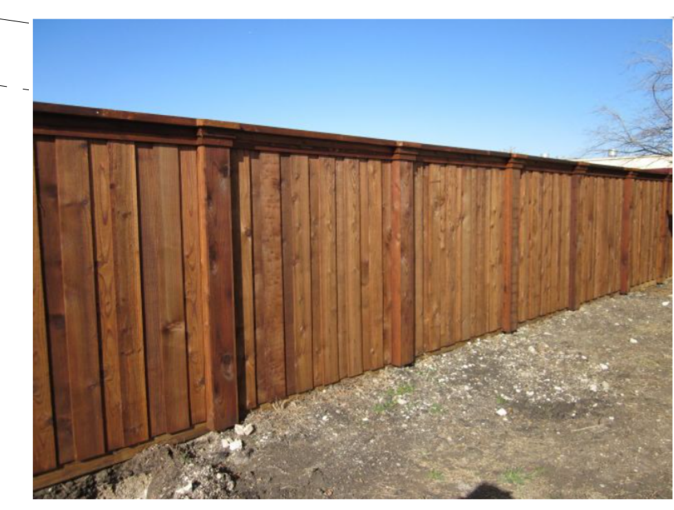
6' WOOD FENCE WITH GAPS COVERED AS SHOWN IN PICTURE
