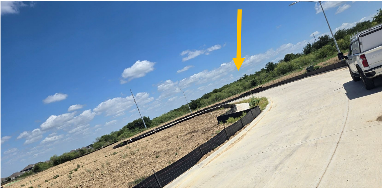
Figure 1: Site Photo taken by staff on 2/24/25; view looking north to the site
