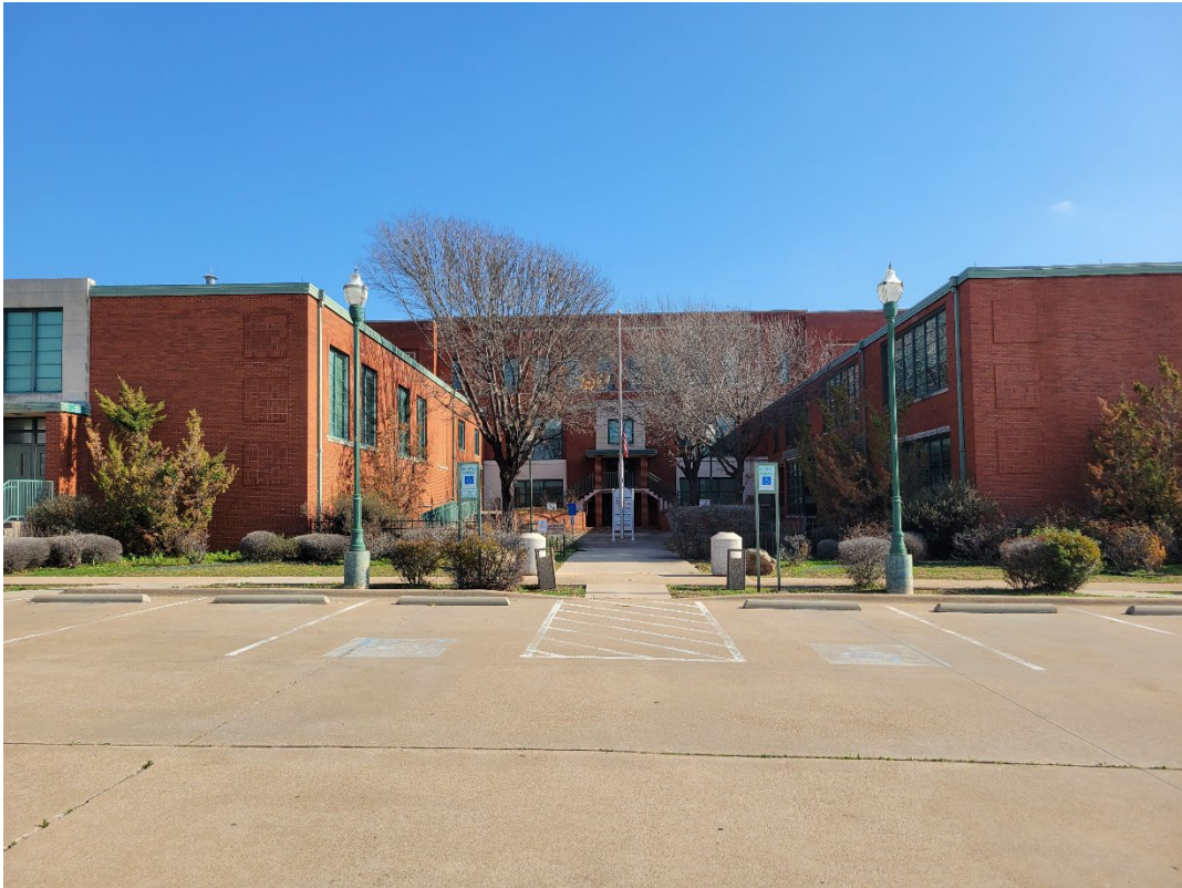
Figure 9 Front view of 1201 E 13 th St
