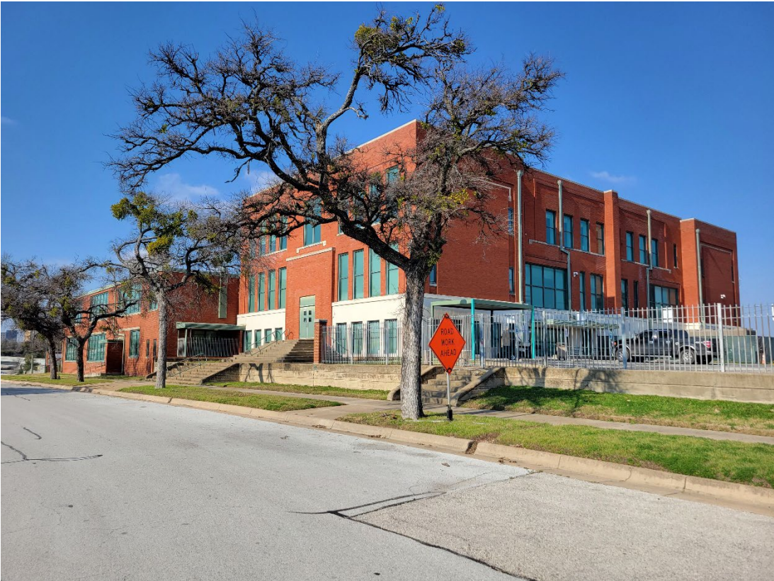
Figure 12 View of southeast corner
