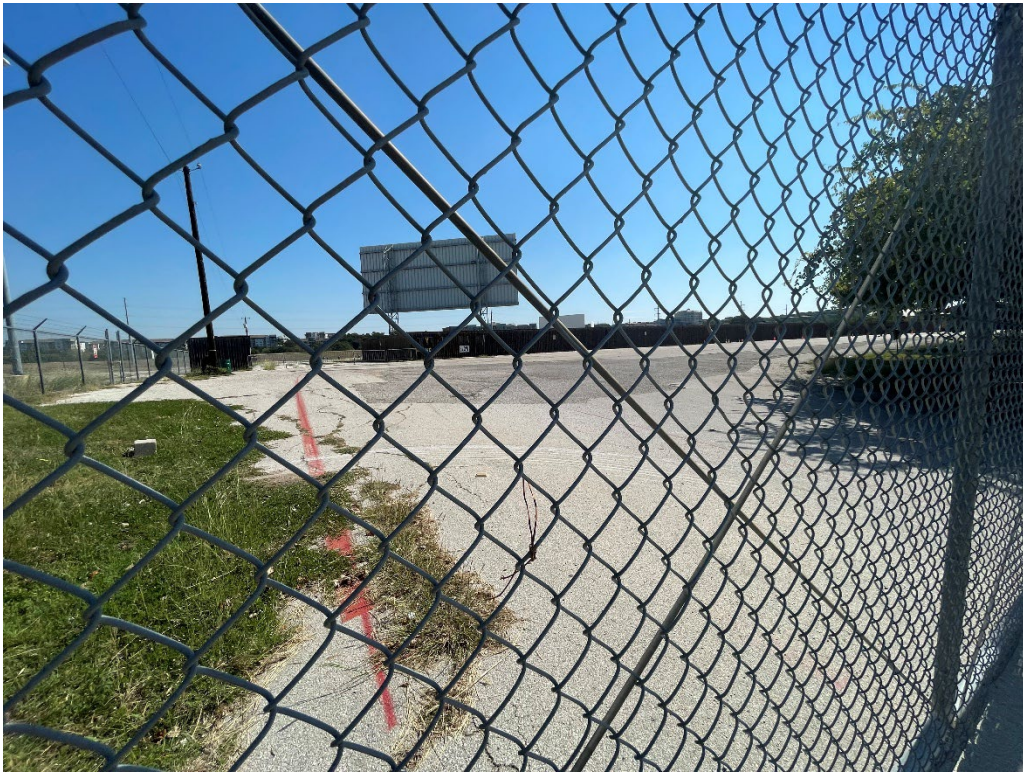
Figure 8 Site photo looking southeast into the drive-in theatre property
