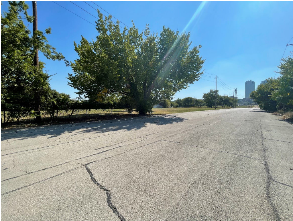
Figure 5 Site photo looking Southeast along Commerce
