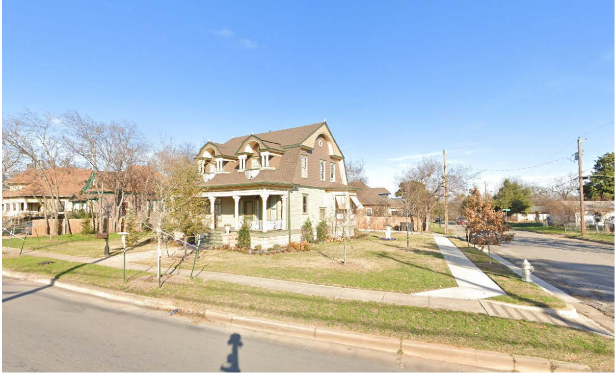
Fig. 3 – Talbott-Wall House at its new location at 1102 Samuels Avenue.
