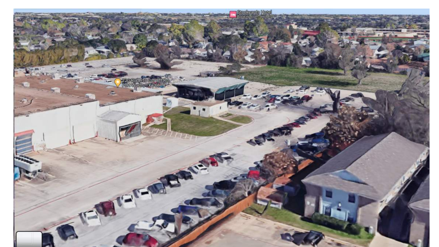
VIEW FROM SW BEFORE
