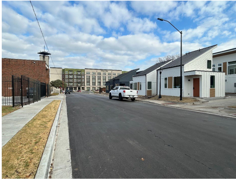
Figure 6. Site Photos showing Casita buildings along Galveston
