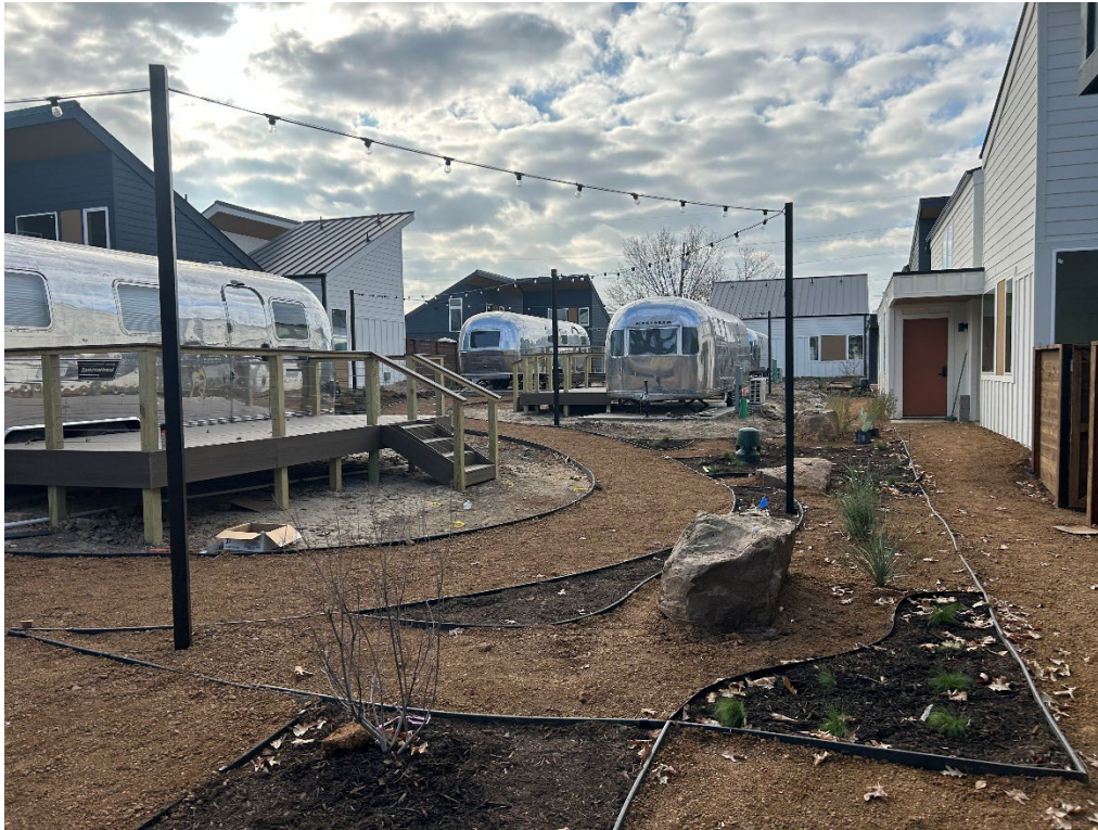
Figure 2. Site Photo showing recreational vehicles on the site during construction
