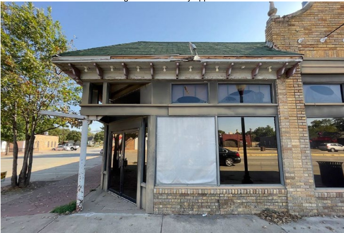
Figure 11. Photo by applicant
