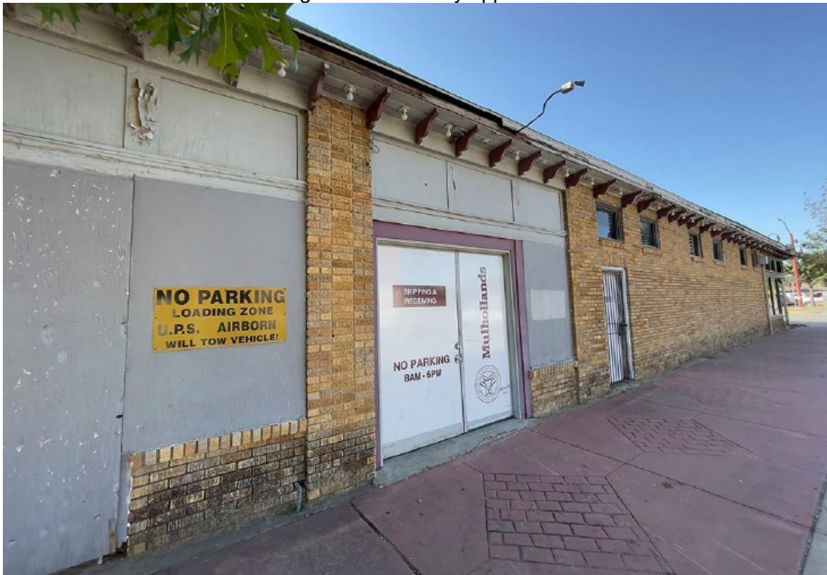
Figure 13. Photo by applicant
