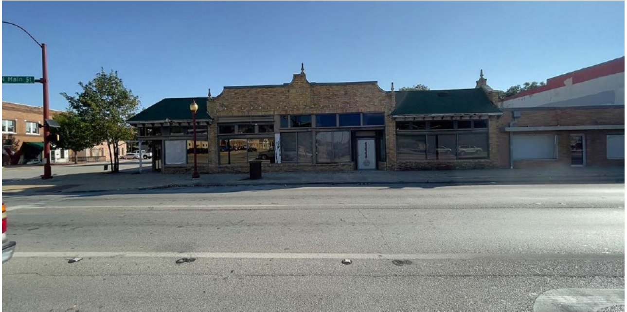
Figure 8. Photo by applicant
