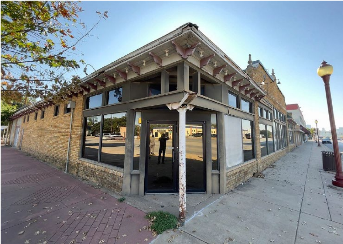
Figure 12. Photo by applicant
