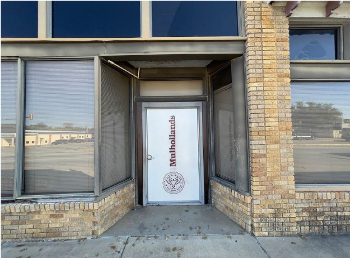
Figure 10. Photo by applicant.
