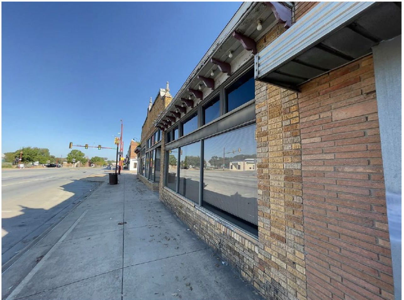
Figure 9. Photo by applicant
