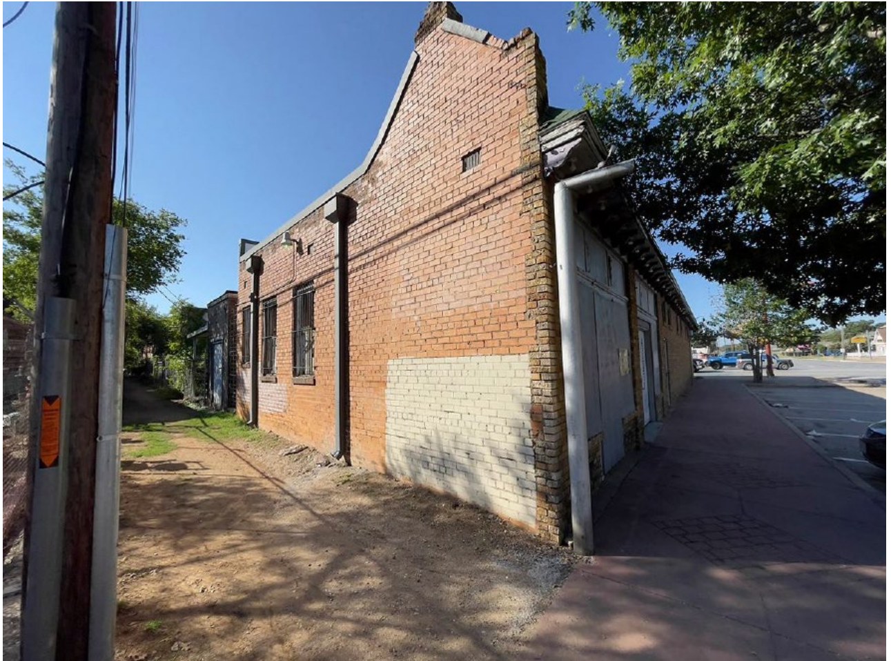
Figure 14. Photo by applicant.
