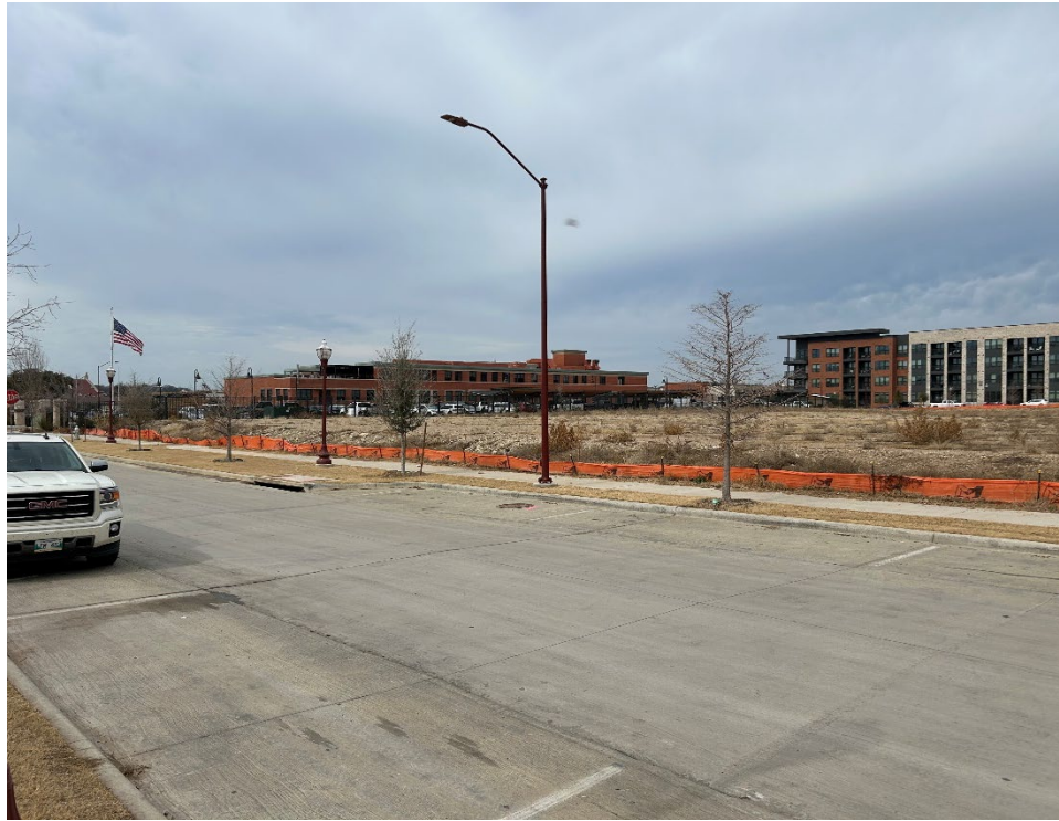
Figure 1. Site Photo from SW of subject site, Armour Building in background (taken 2.10.2026)
