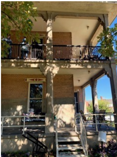
Fig. 7 – Left elevation. Note wraparound porch, concrete columns with decorative faux-concrete brackets.
