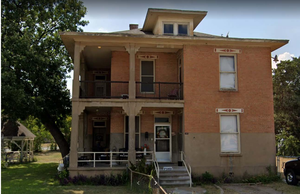
Fig. 6 – Front façade. Note concrete cladding and porch posts, metal handrails, and decorative elements above 1/1 wood windows. Also note wide, overhanging eaves and dormer, which are indicative of the Italianate and Empire styles.
