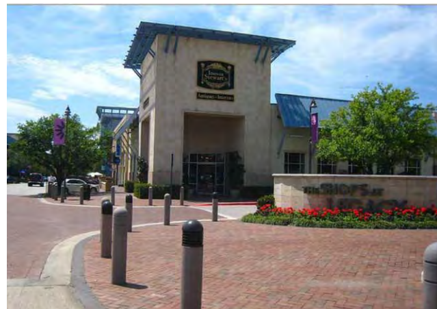
A corner building with architectural elements at a pedestrian scale.
