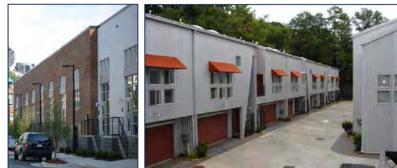
Industrial Arts building organization
