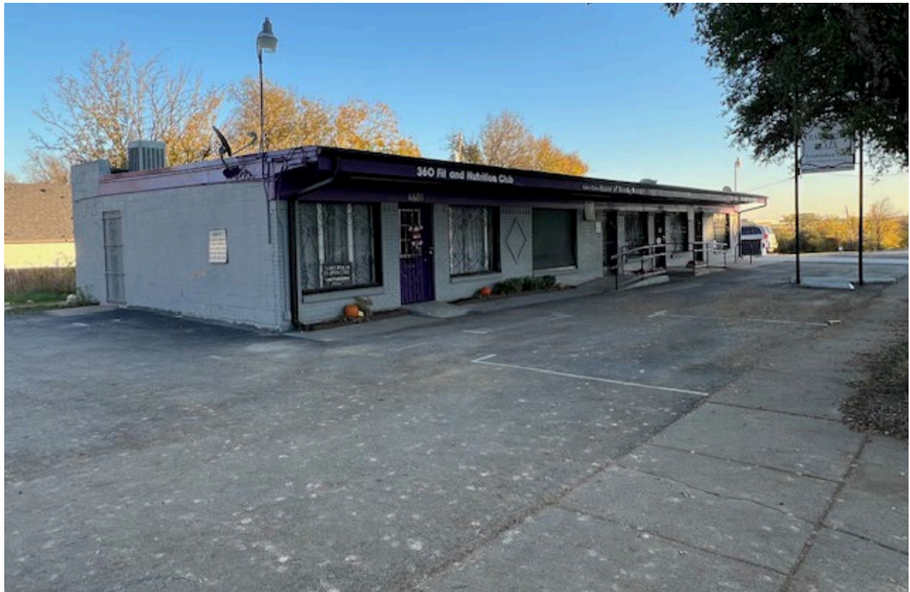
Fig. 3 – Showing primary structure. The original windows and doors appear to be modified/replaced; it also appears that bars were added to the windows. The original brick siding was painted, additional signage was also added to the façade along the roofline
